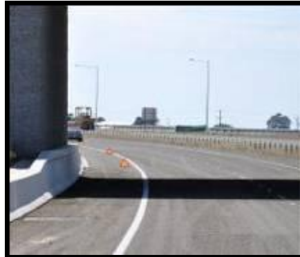
The view for traffic is obscured by the bridge.
